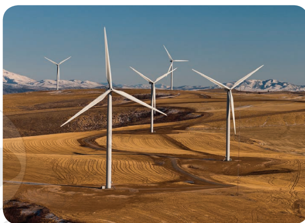
Fig. 17.8 Windmills for electricity generation
